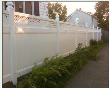
Board and Lattice Gothic tops
